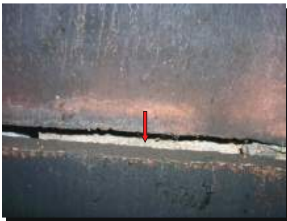
(2) Gap between flue liners as viewed through electronic scanner.
