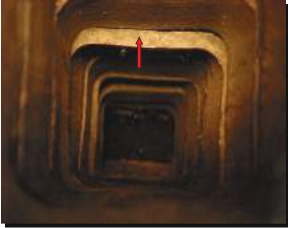
(1) Misaligned flue liners.
