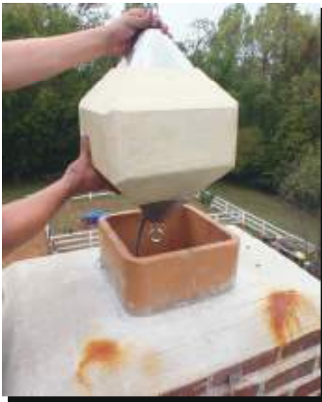
(1) A closed-cell applicator with an internal vibrator is installed in the top of the flue and winched down to the base of the flue.
