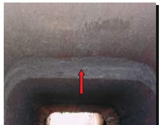
1" off-set between flue liners solidly filled.
