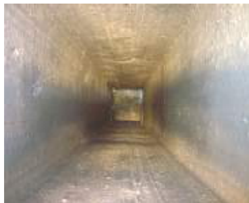
Fractured flue liners completely resurfaced.
