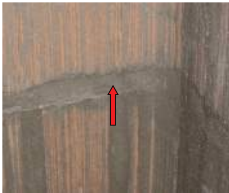
1" open mortar joint solidly filled.
