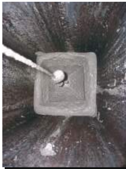
(2) The FireGuard material is then blended and poured on top of the vibrating applicator as it is winched up the flue. The applicator is drawn up and down the flue for multiple passes.
