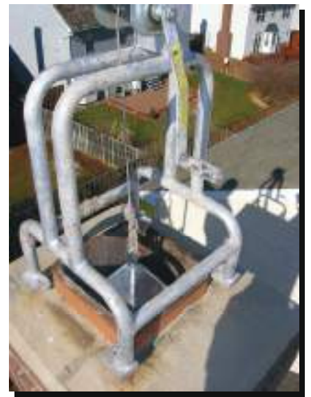
(3) Top winch is used to pull the vibrating applicator up the flue.
