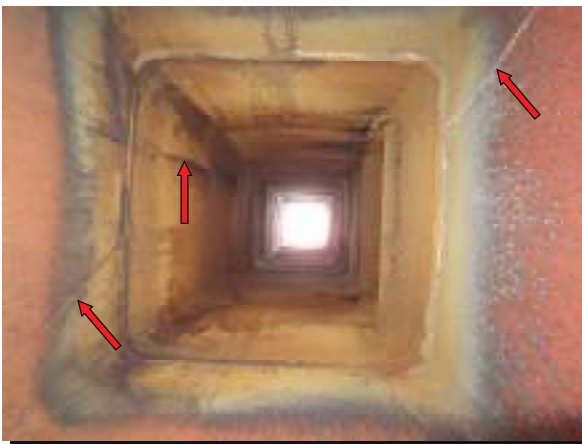
(3) Fractured flue liners.
